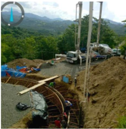
Buenavista Water District Reservoir Tank
