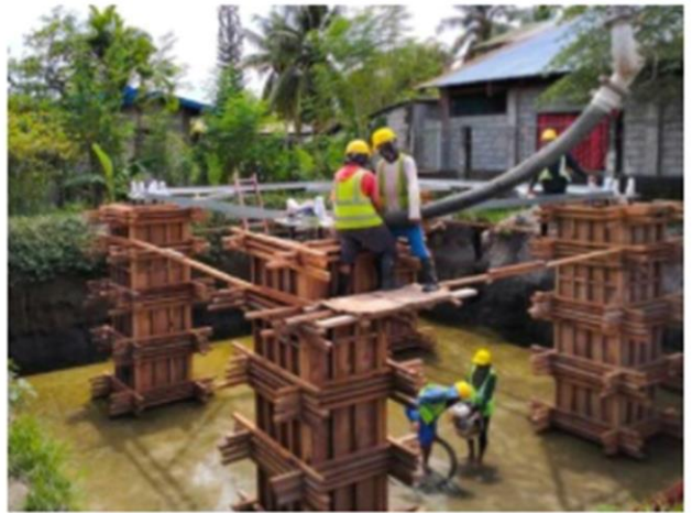
Dito Telecommunity Towers
